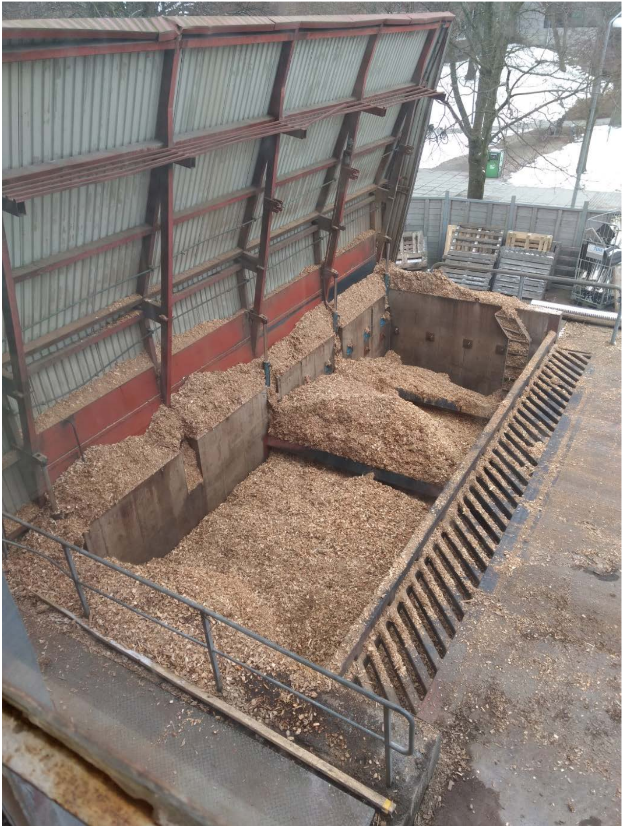
Woodchips for the boilers producing heat and electricity
